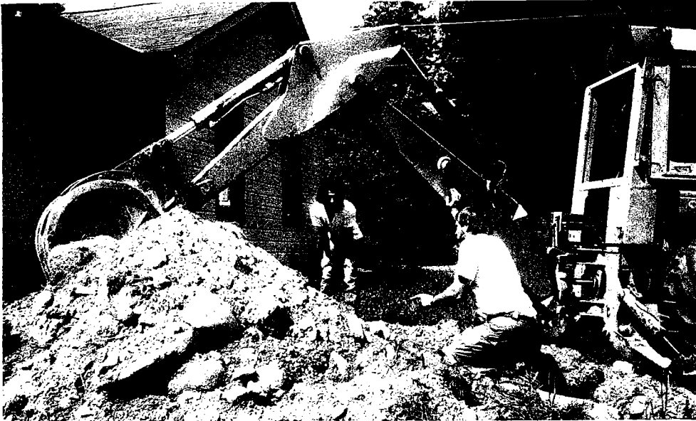
Rodney Sage, installing the septic system with help from Jeremiah Adams
